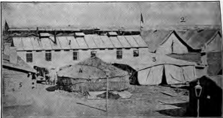
FIG. 207.—Livonian field hospital, Mukden, Manchuria. 1, portable Doecker pavilion; 2, large Russian hospital tents; 3, tortoise tent or ridge pole (system Lefebvre); 4, Mongolian felt tent; 5, small frame barrack for personnel.
